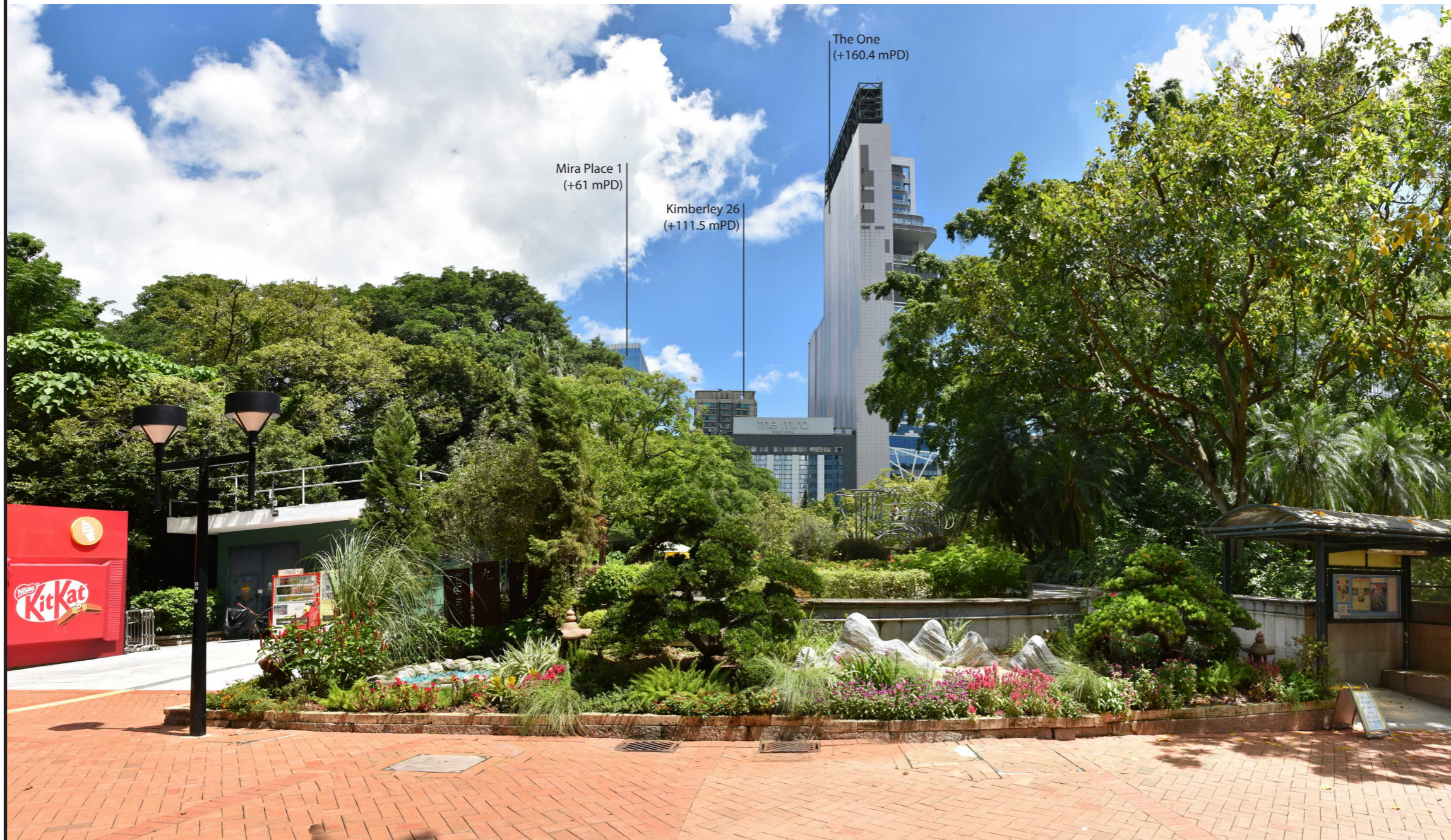
Vantage Point 04: View looking east from Kowloon Park (Existing Situation)
